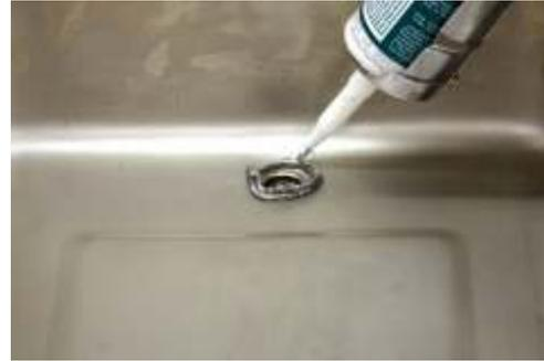
8. Press Drain Cover onto sealant firmly. Then clean any excess sealant from around the Drain Cover. Allow sufficient time to cure (at least 12 hours).
