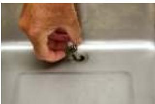
7. Liberally place silicone sealant (recommend DOW CORNING RTV sealant 732) around the edge of the drain.
